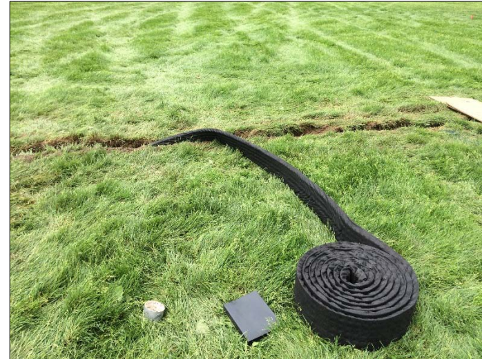
Trench & Slit Drain Installation
