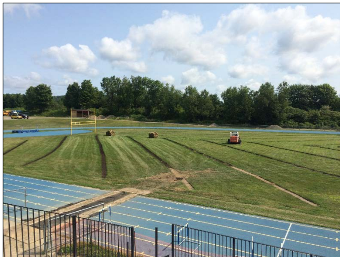
New Sod Over Slit Drains
