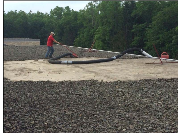
Removing the Ballast
