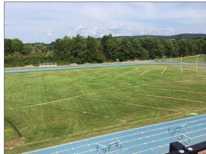
New Sod Over Slit Drains
