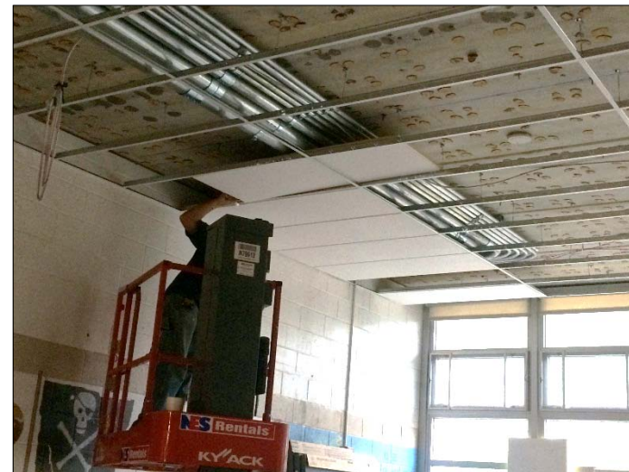
New Ceiling Tile Installed
