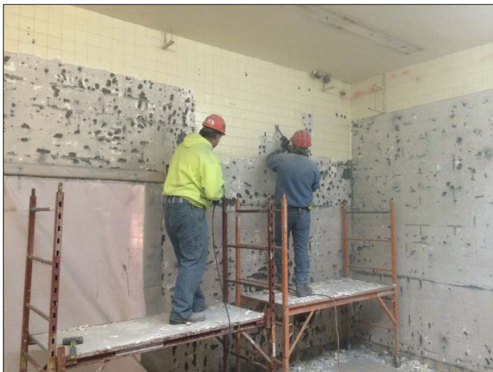
Removing Wall Tile
