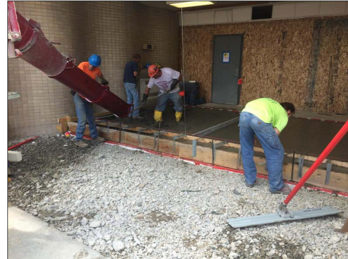
Removing Old Sidewalk New Foundation at Doorway/Vestibule Entrance
