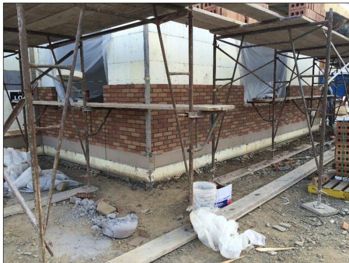
Exterior Brick Applied
