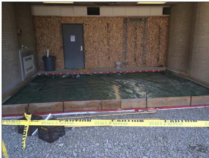
Moisture Barrier & Concrete Cure
