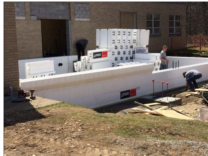
Walls Going Up (Insulated Concrete Forms)
