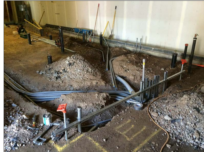
All New Utilities Under Slab
