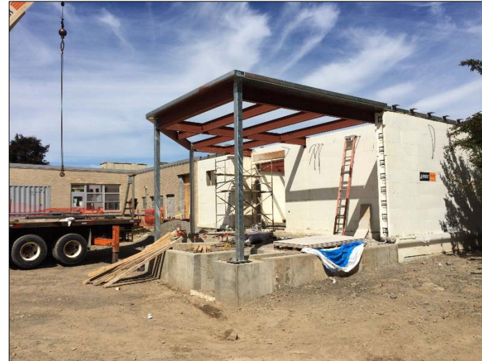
New Structural Roof Deck
