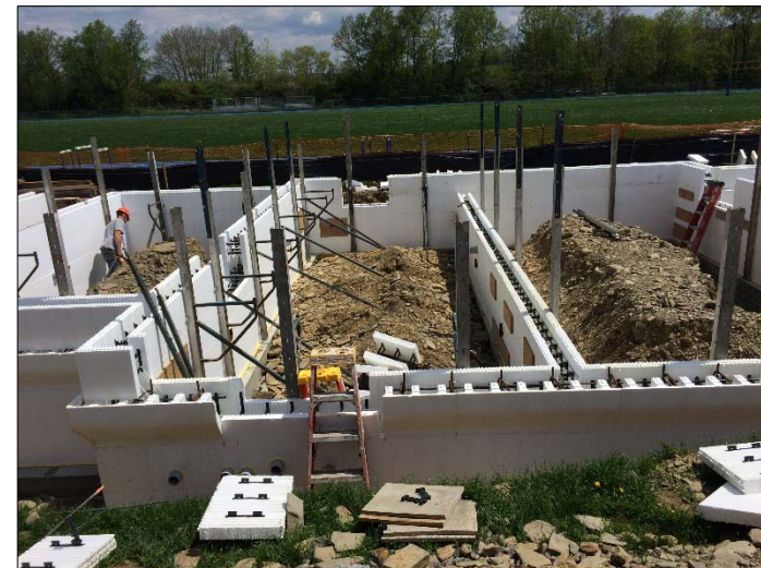
Walls Going Up (Insulated Concrete Forms)
