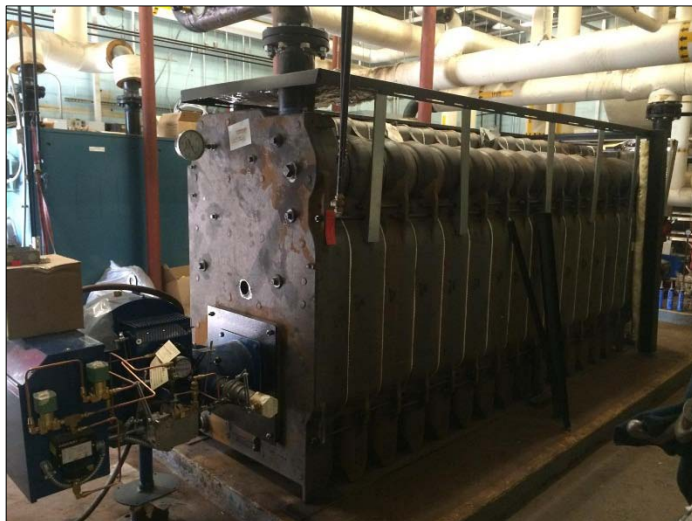
Installation of New Sectional Boiler
