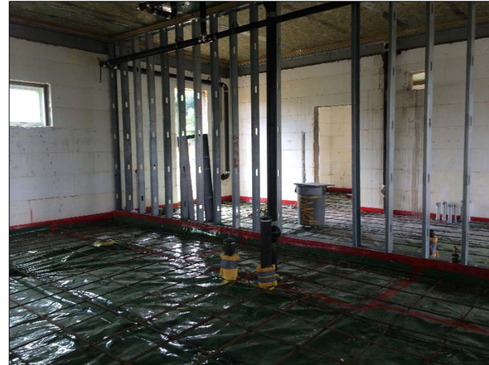
Framing Walls and Floor Prep (Moisture Barrier)
