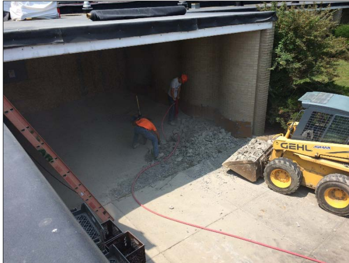
Removing Old Sidewalk New Foundation at Doorway/Vestibule Entrance
