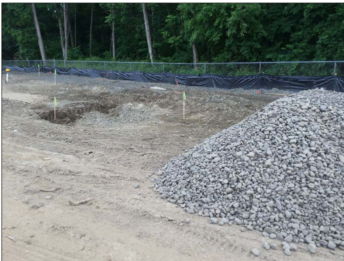
Stone Delivery For Undercuts
