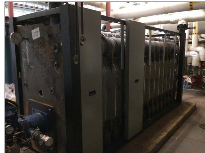
Installation of New Sectional Boiler
