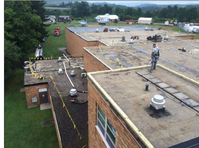
Wood Blocking at Roof Edge
